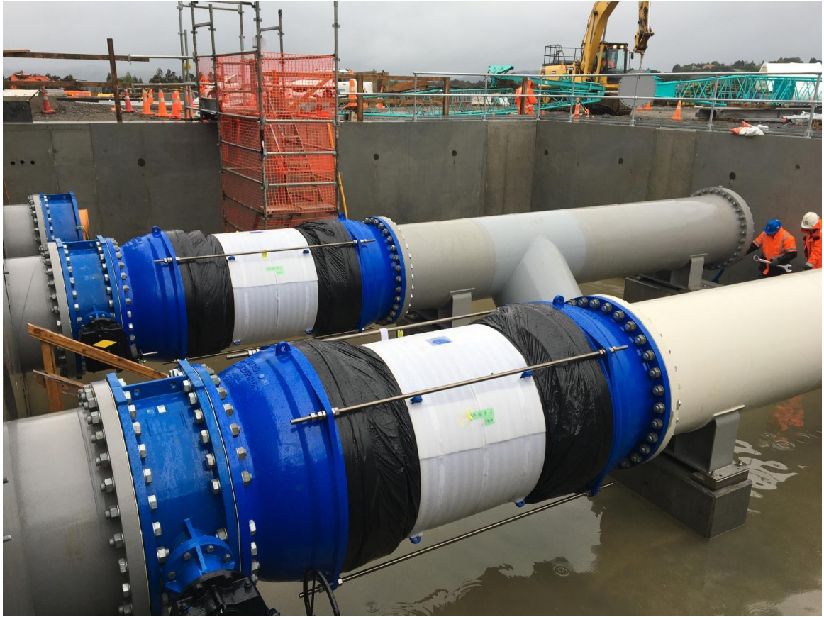
Completed Valves and Dismantling joints installed with Allied Fastenings Dressing Sets
